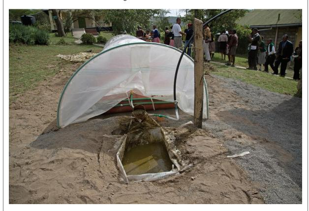
The solution might, in part, come from the use of biogas digesters (shown above). The biogas digesters use any bio-degradable material e.g. animal or human waste, garden weeds and kitchen waste. They are highly efficient, have a life span of over 10 years and come in varying sizes.
