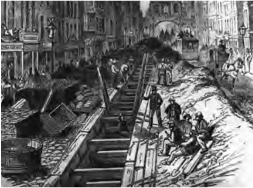
The construction of sewers in London, 1844.
